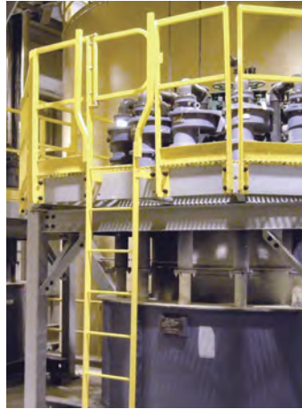
Raised platform with protected guardrail.
